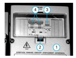
If the 230 V system is electrically defective or overloaded, switch the fuses (4) in the automatic circuit breaker (1) with earth leakage protection to the "OFF" position.
