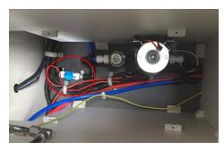
Drain valve of the fresh water tank
