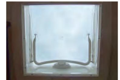
In order to open the skylight, press the release button to unlock the bracket and pull the bracket down. Then pull the bracket towards you to lock it into one of the three opening positions. To close the skylight again, lift the bracket out of the recess, push it forward and slide it over the release button.
