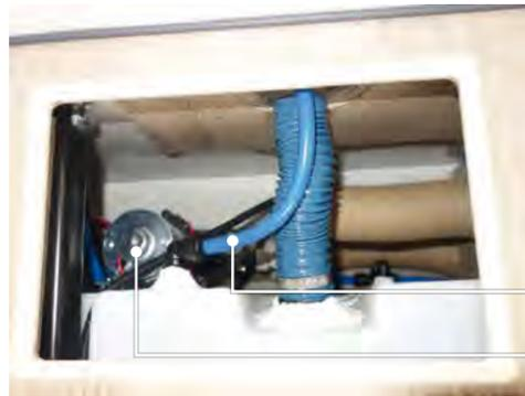
The pump is located under the front bench, next to the fresh water tank.
