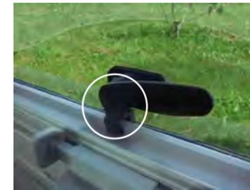
The windows can also remain open in a position for permanent ventilation by inserting the lever into the recess of the window lock.
