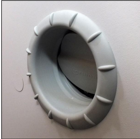
Outlet opening for hot air
