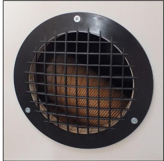
Intake opening for circulating air
